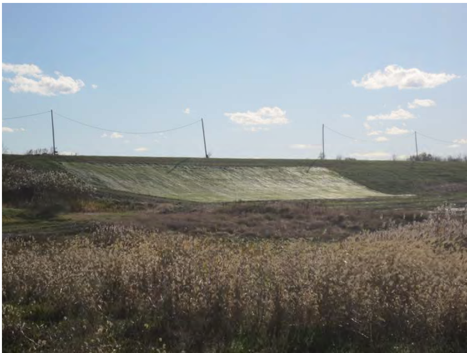
Figure I.2. Photo of 2015 surficial movement area after repairs.
